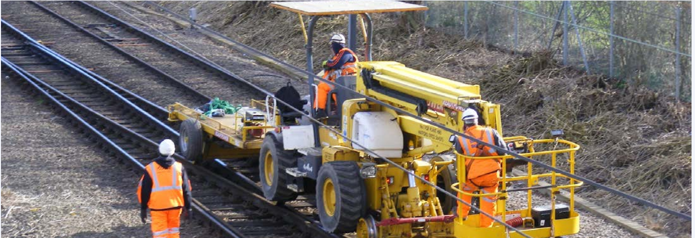
Figure: Overhead line inspection similar to the one undertaken by Ferrous Metals SA
